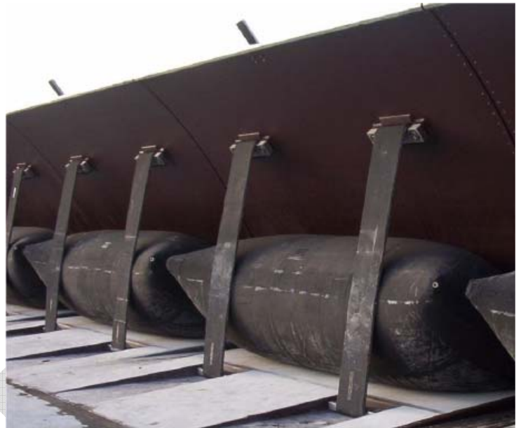
Figure 7. An Obermeyer Gate installation Showing Steel Panels, Air Bladders and Stabilizers
