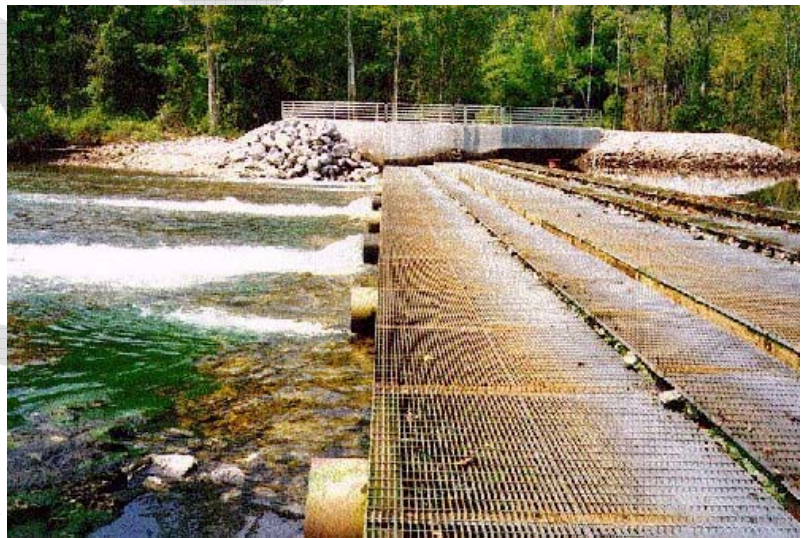
Figure 8. TVA Norris Weir's Stepped Weir Deck
