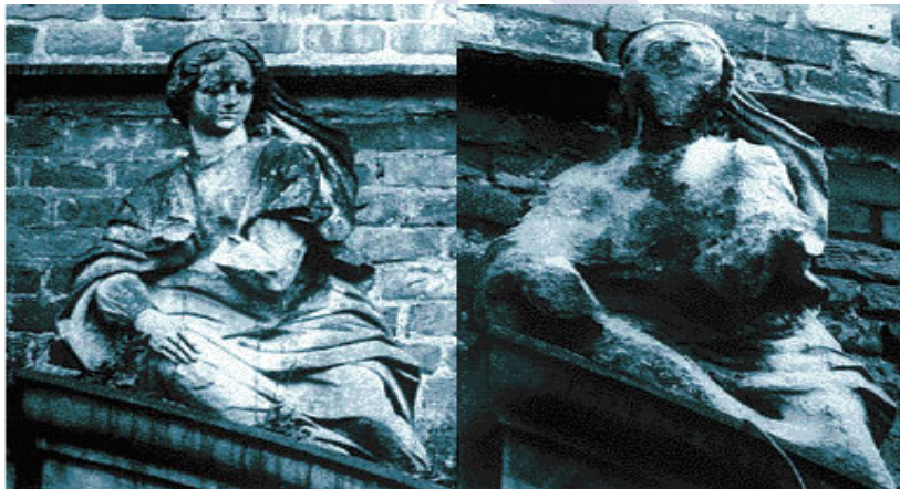
How acid rain affects stonework. The picture on the left was taken in 1908. The picture on the right was taken in 1968
