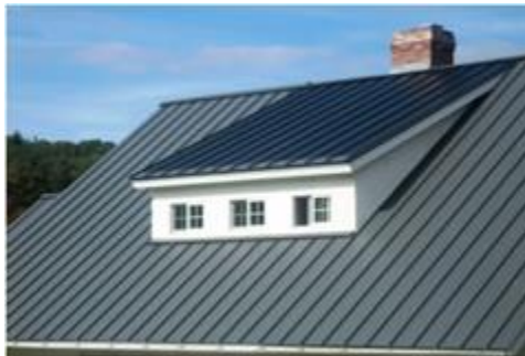
Figure 19-11: Building-Integrated Solar Energy System
